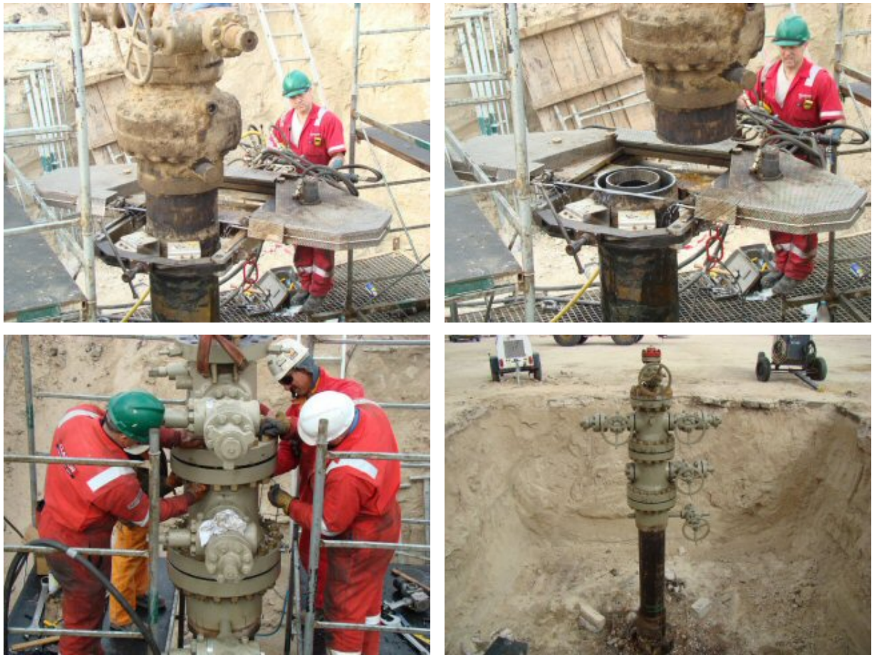
Figure 1: Replacement of a wellhead due to deterioration & environmental degradation
